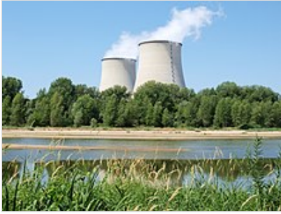
Belleville Nuclear Power Plant.
