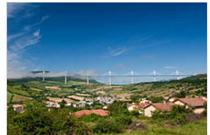
Millau Viaduct is the tallest bridge in the world . [208]
