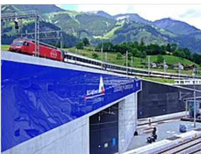
Entrance of the new Lötschberg Base Tunnel , the third-longest railway tunnel in the world, under the old Lötschberg railway line . It was the first completed tunnel of the greater project NRLA .
