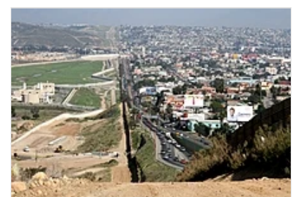
The Mexico–United States border wall between San Diego (left) and Tijuana (right)
