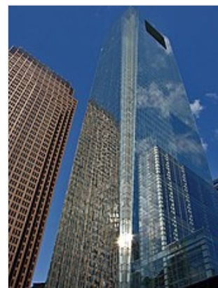
Comcast Center in Philadelphia , headquarters of Comcast , one of the world's largest telecommunications companies and media conglomerates
